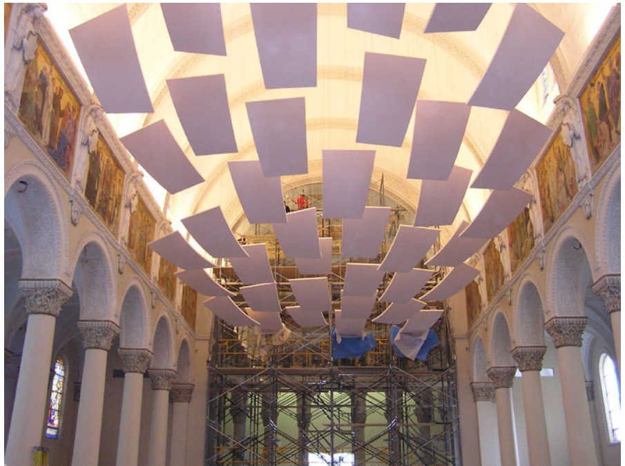
"In Construction - raising the glass partitions"
