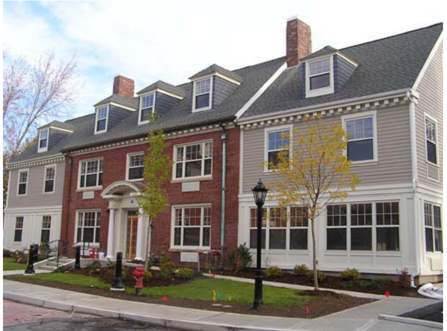
"Seton Manor" Hospice Care Building
