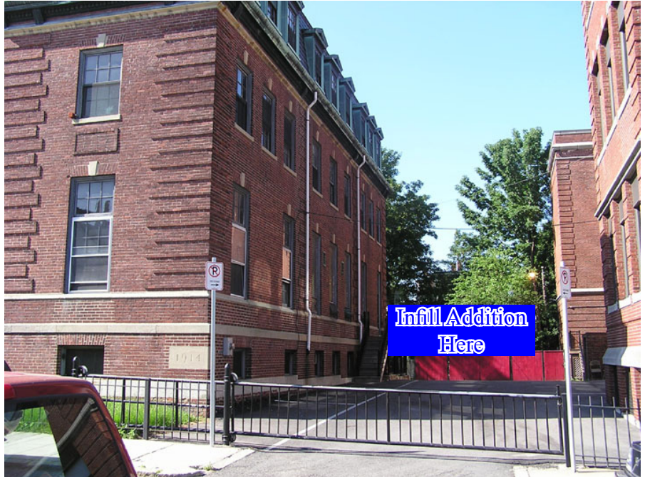
Convent on left, existing high school on right
