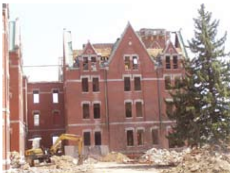
Kirkbride Building "Under Rehab"
