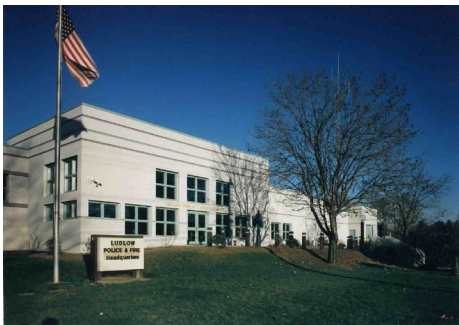
Police and Fire Fighting Facility Ludlow, Massachusetts
