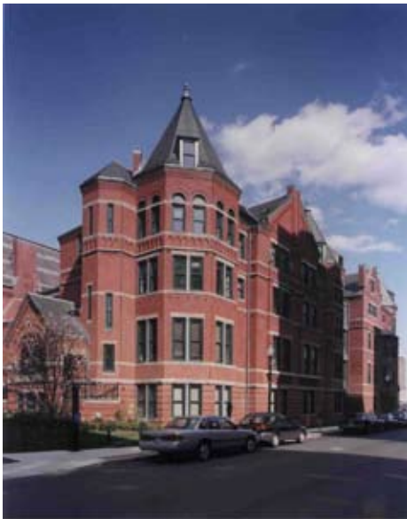
Boston University's Talbot Building - Boston, Massachusetts Photo by Peter Vanderwarker
