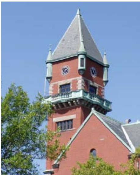
Leventhal-Sidman Clock Tower Repair Newton, Massachusetts
