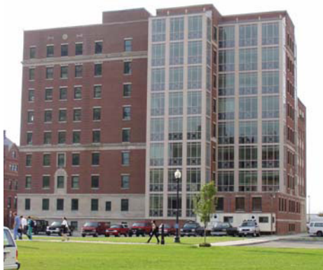
Surgical Building - 85 East Concord Street
