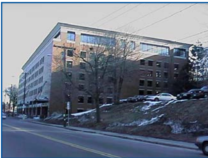
Tufts University Parking Garage and Offices (Seven-stories) Filigree Wide Slab Floor System
